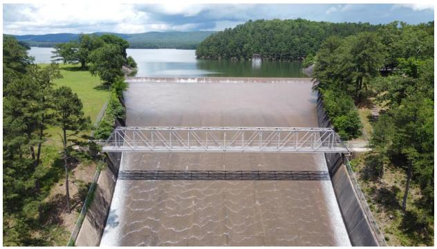
Figure 4. Improvements to the spillway at Lake Winona is one of the nominated projects in the green bond, which will increase the resiliency of the system, decrease contaminants into the system, and improve functionality.
