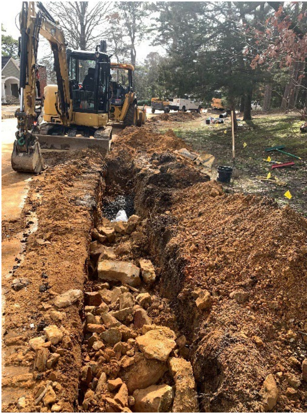
Severe, rocky soil conditions have been encountered on this project.
