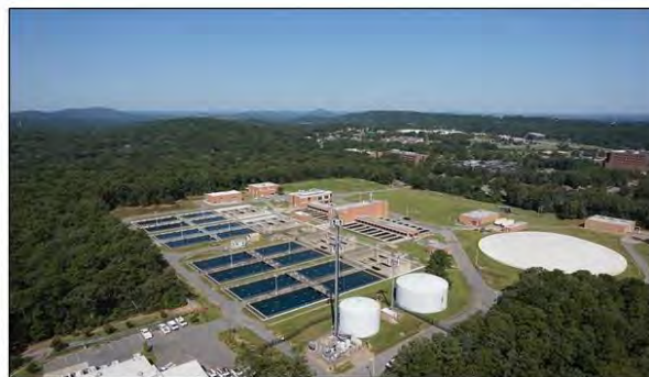
2017 aerial photo of the Wilson Plant.
