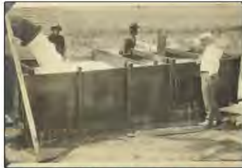
Treatment Water Well E – April 1925 – Arkansas Water Company employees try to figure out how to stop the leak.
