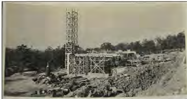
Oct. 29, 1937 – Ozark Point Plant under construction.
