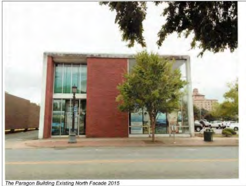
The Paragon Building Existing North Facade 2015
